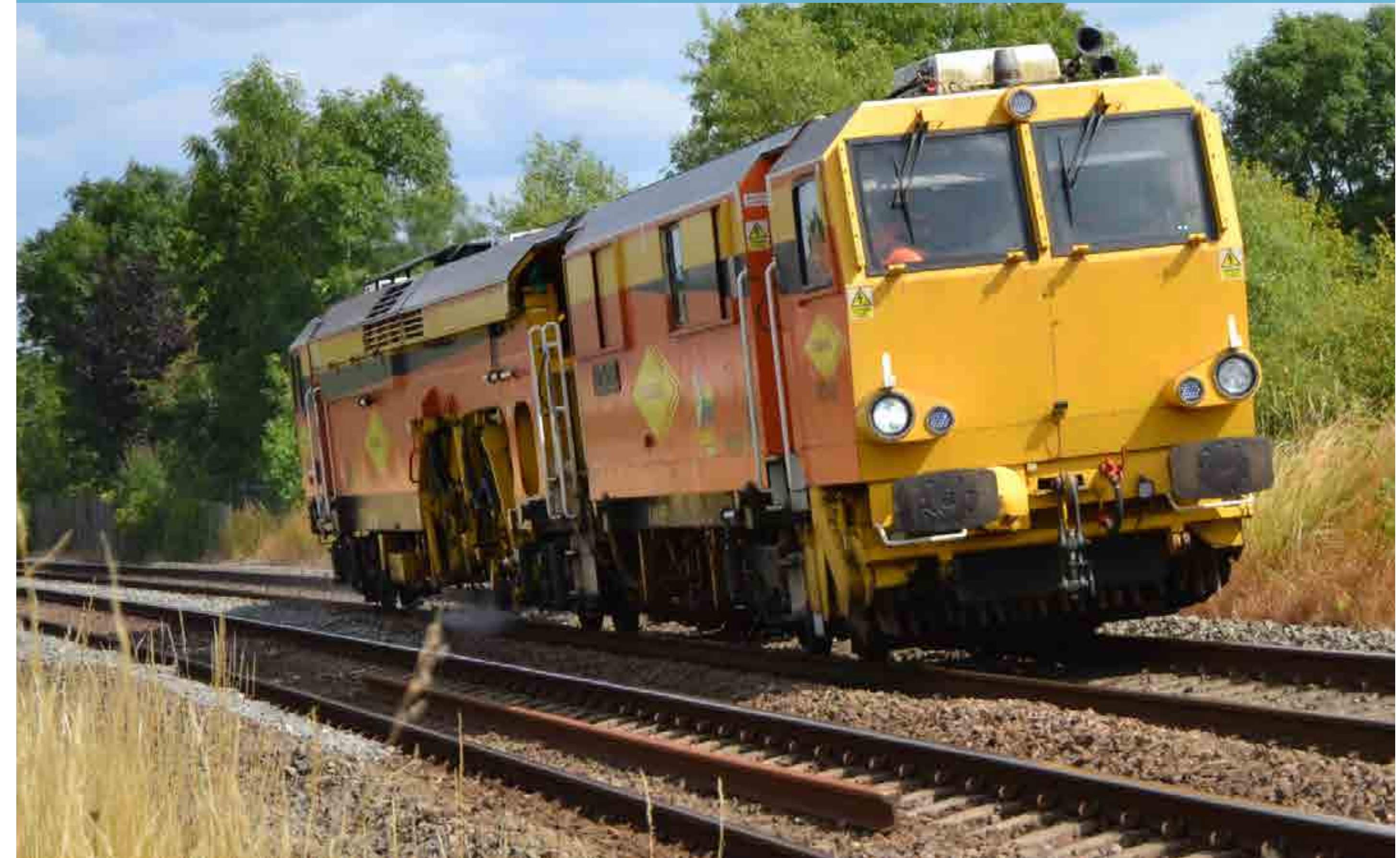
Colas Rail's track machine No. DR75406 working the 6J83 Reading Triangle to Gloucester (Horton Road) passes Purton Lane foot crossing on July 18th. Ken Mumford
