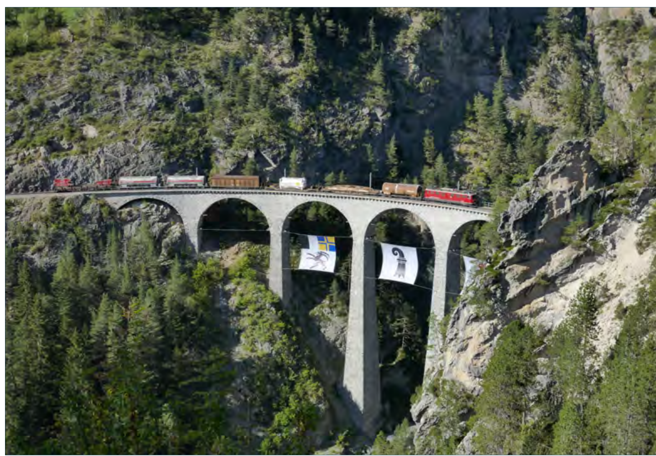
▶ Ge 6/6II No. 704 with a southbound freight is seen crossing the Landwasser Viadukt. Steamsounds
